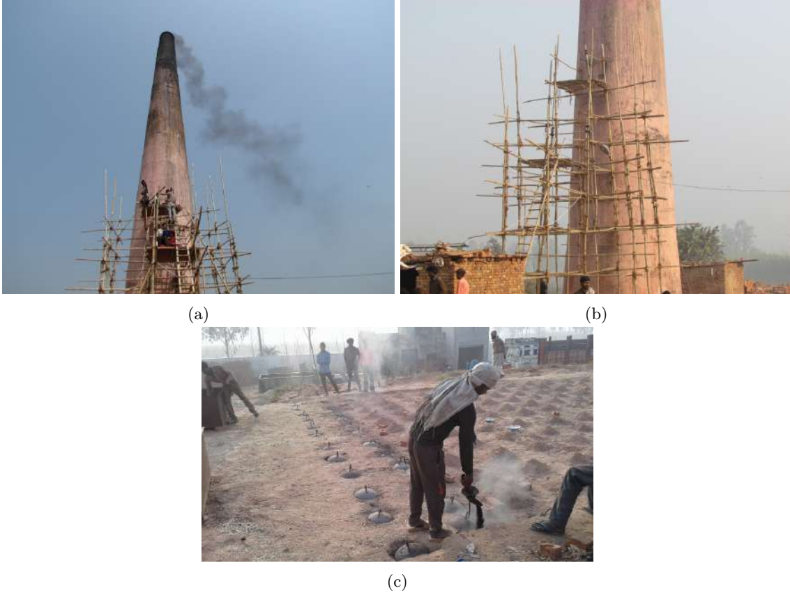
Figure 1: (a) Chimney of BTK measured in India. (b) Scaffolding setup on central stack. (c) Manual coal feeding in BTK.
